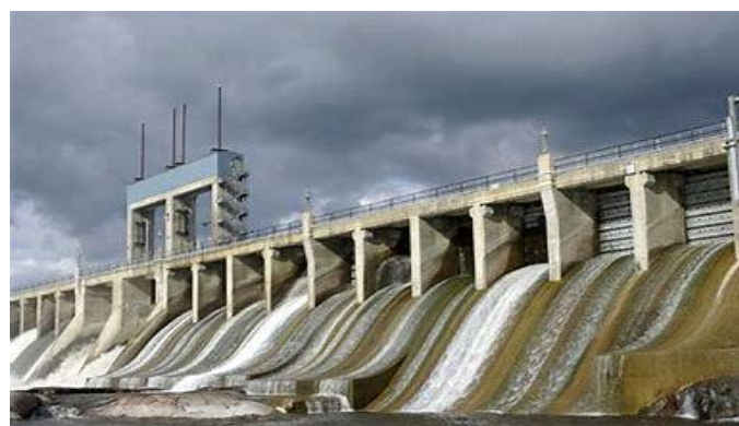
Figure3. Hydro power plants
