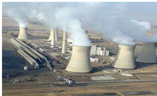
Figure2. Thermal power plant
