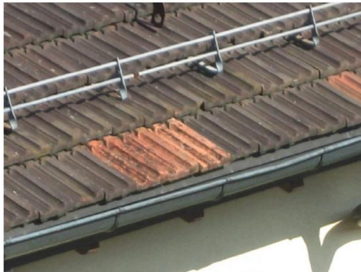
Figure 10. Roof with recently substituted bricks
